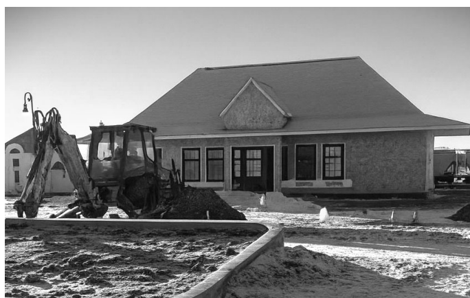
Replica Biggar Station for Brownlee Square under construction, 2025
