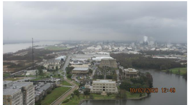
Baton Rouge LA – View from the 34 th storey of the State Capitol building. CN/IC rail yard is on the right side of the Mississippi River shown on the extreme left of the photo.
