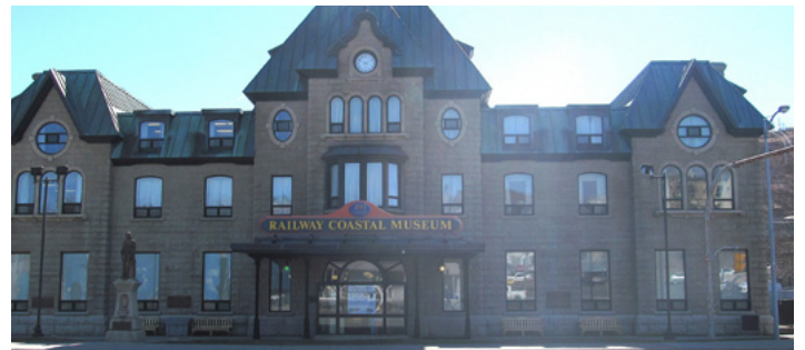
Riverhead Station Railway Coastal Museum
